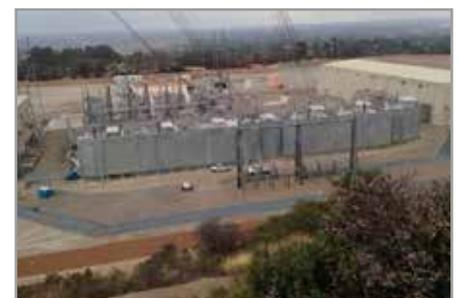
Figure 6. Major US substation protected from hillside by UL 752 Level 8 [2] ballistic fire barriers installed to NFPA 851 [1]
