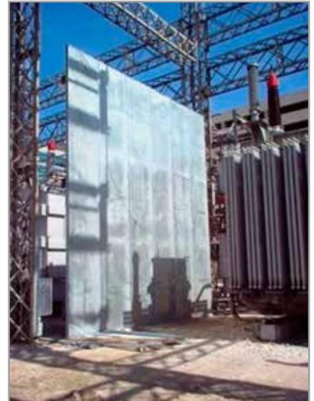
Figure 9. Local CIP using proximity ballistic fire barriers
