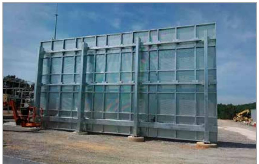
Figure 10. Modular steel fire and impact rated transformer barrier
