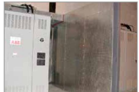
Figure 8. Critical equipment separation wall
