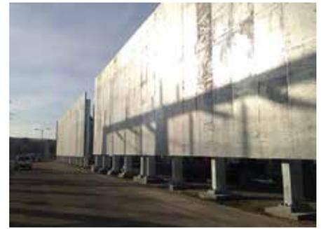
Major US substation protected by UL 752 Level 8 ballistic fire barriers installed to NFPA 851 Line of Sight
