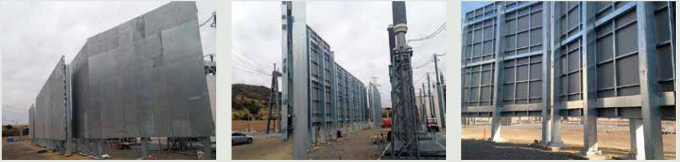
Figure 2. UL 752 tested ballistic fire barriers installed to NFPA 851
